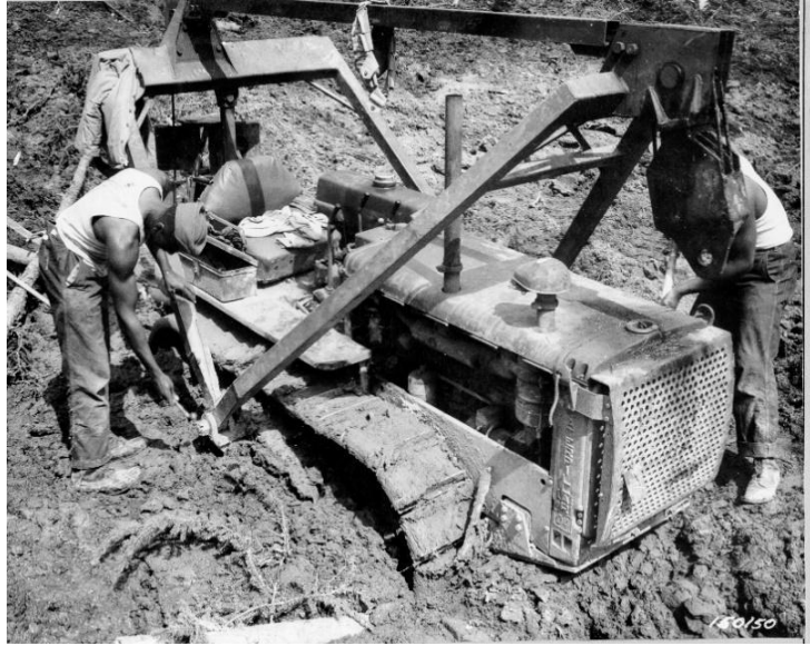
Figure 13: Tracked dozer swallowed up by a muskeg hole. Muskegs sometimes appeared to "swallow" the heavier equipment, then exhibiting thixotropy, when the silty mud mixture "sets up." (Unknown date. Source: US NARA).
